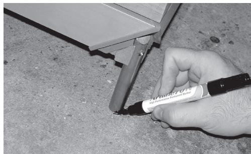
5. Mark the spots where the rods touch the ground. Then move the table or the bench and fit the legs as explained in the Extempore manual.
