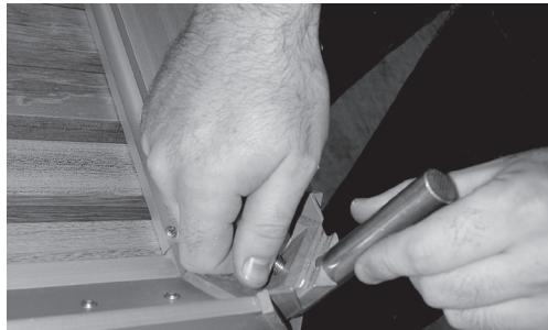
2. Insert the 4 identical stainless steel rods into the holes provided for that purpose.
