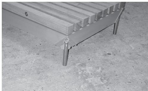
4. Put the table or the bench (without fitting the legs) on the spot where you intend to fasten it to the ground.
