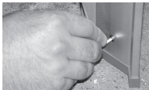
9. Tighten the little screws at the bottom of each leg.
