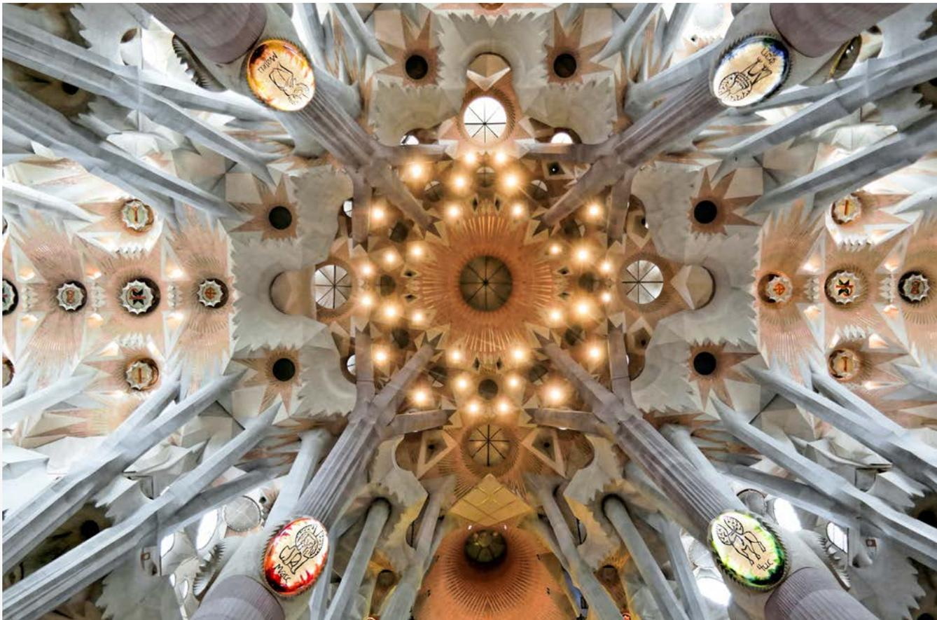
The branching columns of the Nave in the Sagrada Família in Spain mimic a tree where at the intersection of the trunk and the branches, tree knots are used as discrete lighting. It feels like walking in a forest.
