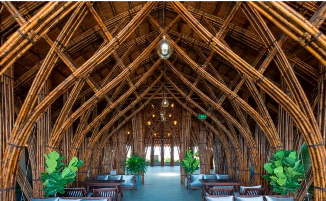
This café in Vietnam is completely made of bamboo. Bamboo grows widely and fast in the region and is a strong material.
