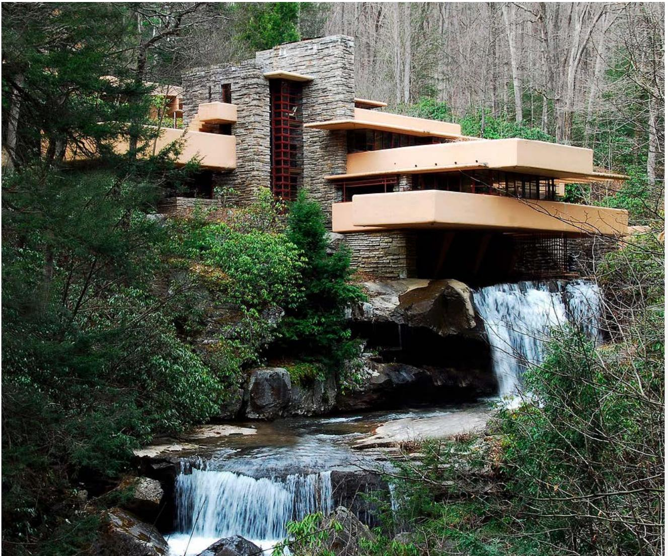
The Falling Water House blends into its natural surroundings as it's built on a waterfall, uses locally sourced sandstone, consists of only two colors and has some original boulders left inside. Even before the term was coined, Wright built one of today's prime examples of biophilic design
